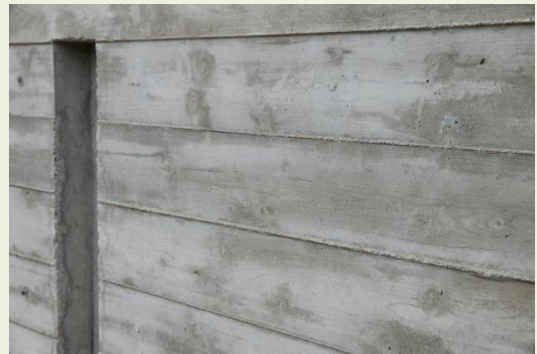
Board Formed Concrete
